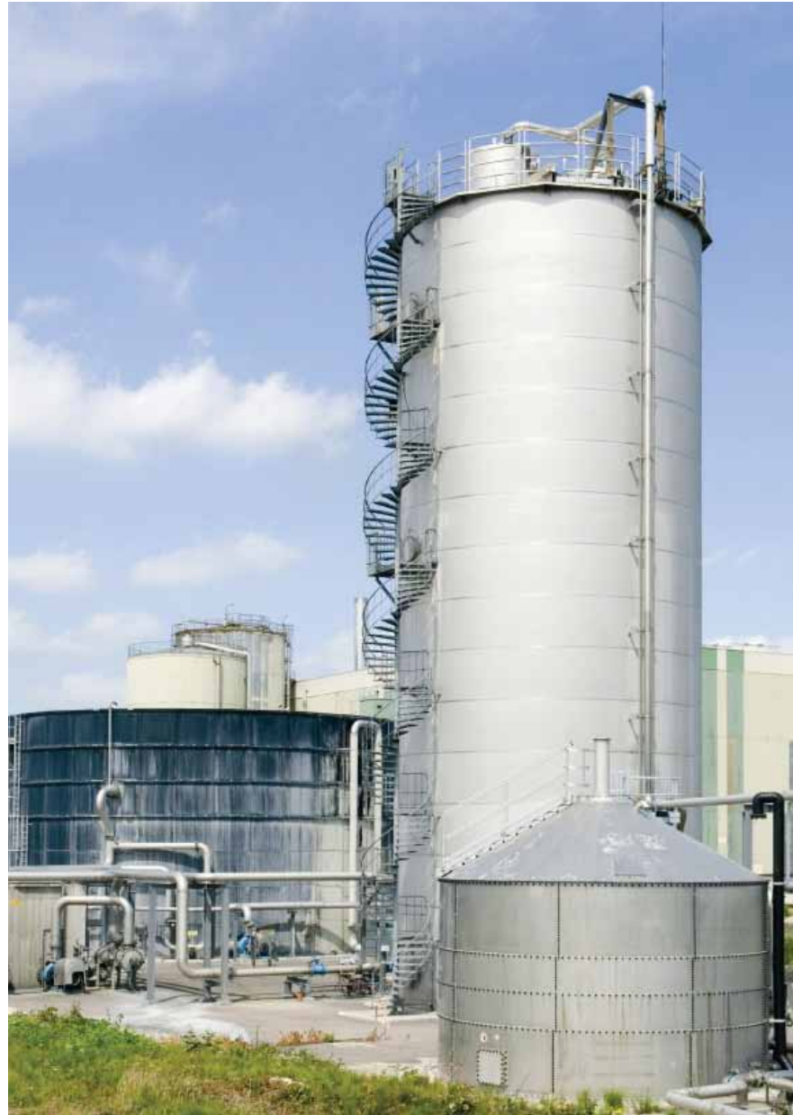
Capstone microturbines running on methane gas generate electricity and hot water for this paper mill in France.
